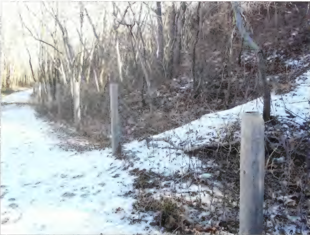
Figure 5.73. View looking northeast along interior trail, the Mortar Battery. In order to protect the historic earthwork, woody vegetation greater than four-inches diameter at breast height should be selectively removed (Olmsted Center, January 2009).
